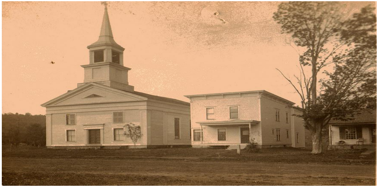
The Post and beam frame of this church rests on massive granite slabs. One story plus attic and steeple. Built in the Greek Revival style, this structure retains the exterior appearance of a typical Greek Revival Church, with a
